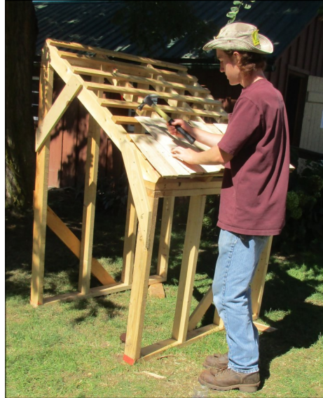
A group of misfits, as they call themselves, got together to demonstrate how to make shake shingles, the most popular roof material in the 1800's. Ben Deuschle and Lucas Drever
